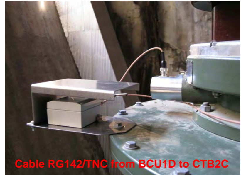
BA7 installed to bushing test tap
